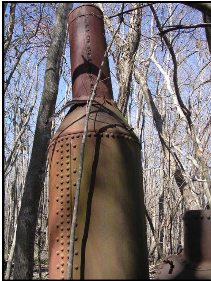
FIGURE B.17. Vertical boiler (photo by author 2007).
