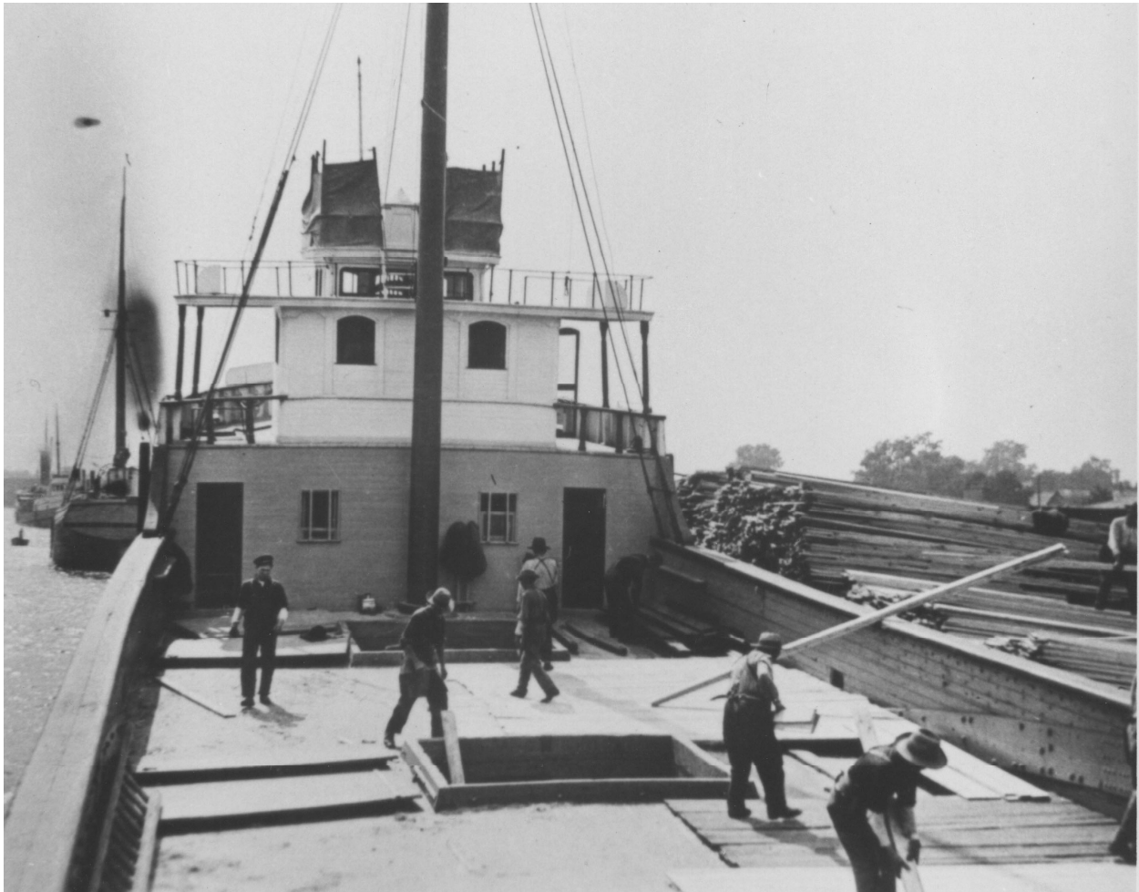
FIGURE 2.5: Lumber shovers filling the hold of a steam barge (Courtesy of the C. Patrick Labadie Collection, Alpena Public Library, Alpena, Michigan).
