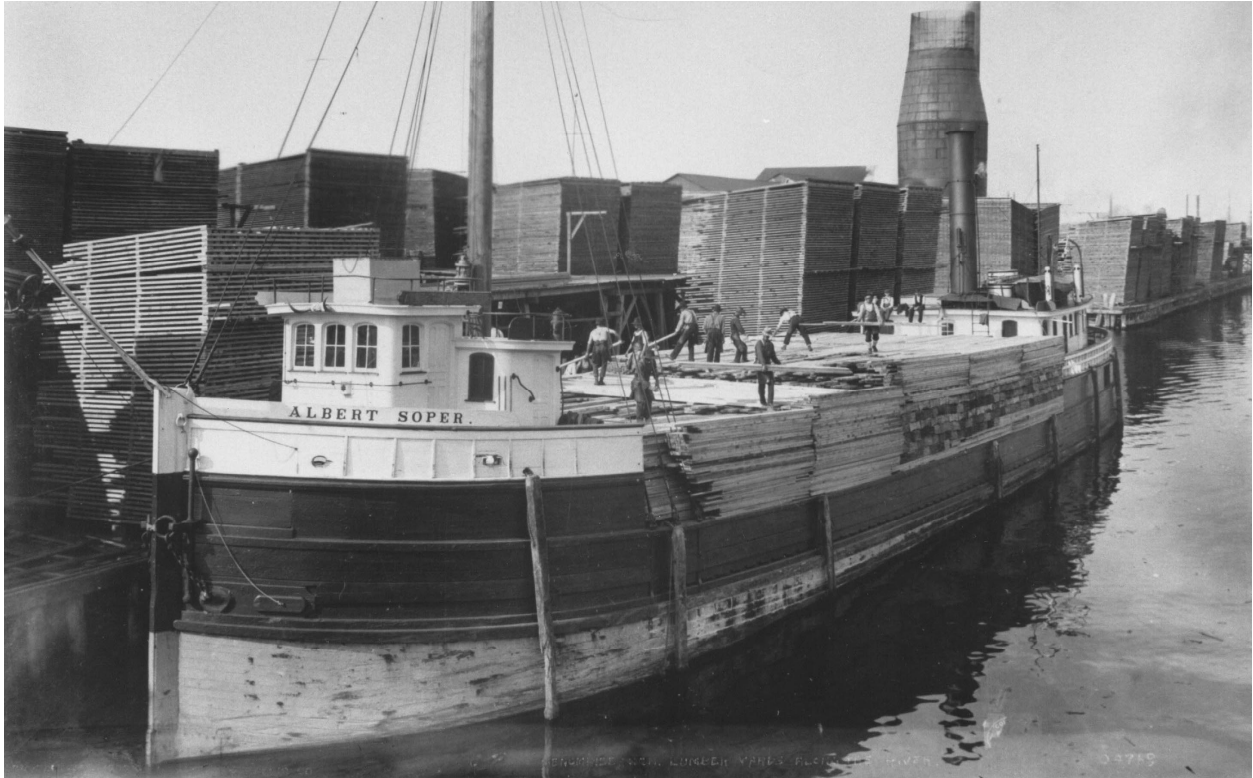
FIGURE 2.6: Lumber Shovers at work. Note how high the cargo is loaded above the deck (Courtesy of the C. Patrick Labadie Collection, Alpena Public Library, Alpena, Michigan).
