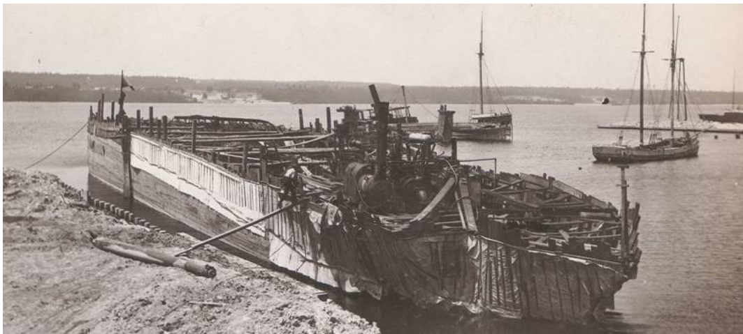
FIGURE 5.4: Joys could possibly be the vessel located directly behind City of Glasgow , pictured in the forefront. City of Glasgow had burned in 1907 after Joys had been abandoned as a breakwater. Note the fore and aft configuration of the vessel, which suggests that it is a steambarge, and the burned condition of the hull (Courtesy the Door County Maritime Museum, Sturgeon Bay, Wisconsin).
