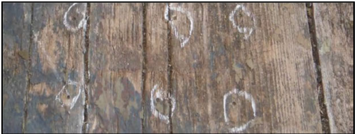
Figure 47. Fastener holes in the hull planking (circled with chalk) associated with stanchion braces in the stern. (Photo by Ryan Bradley, 2013).
