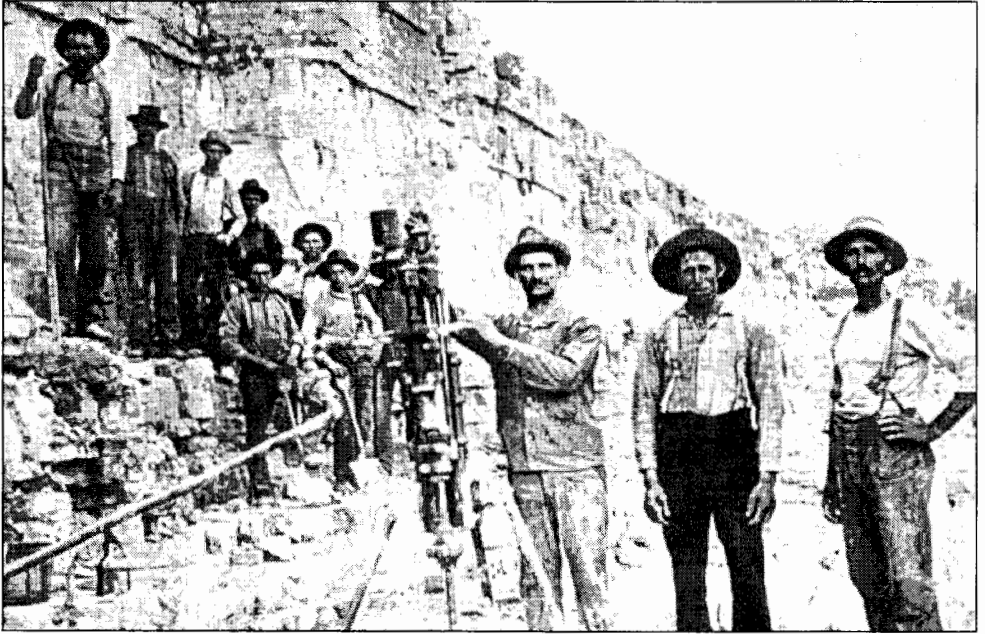
Figure 4. Dolomite Drilling Crew on a limestone shelf. Note the pneumatic drill.
