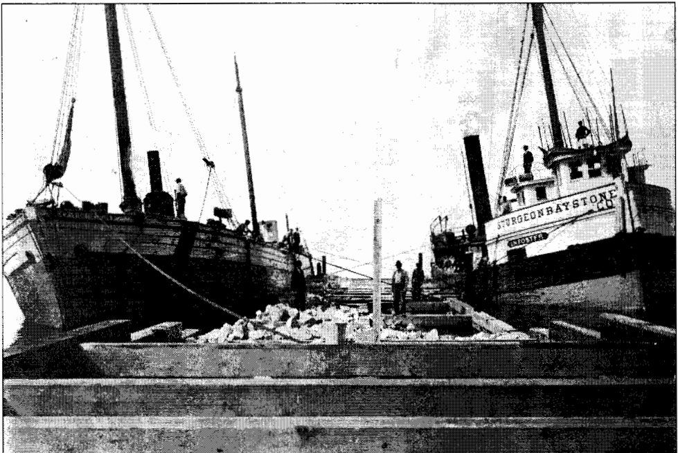
Figure 7. The Oak Leaf and her escort the I.N. Foster unloading stone at a crib pier. Note the donkey boiler on the fore deck of Oak Leaf , and small cabin on the after deck.
