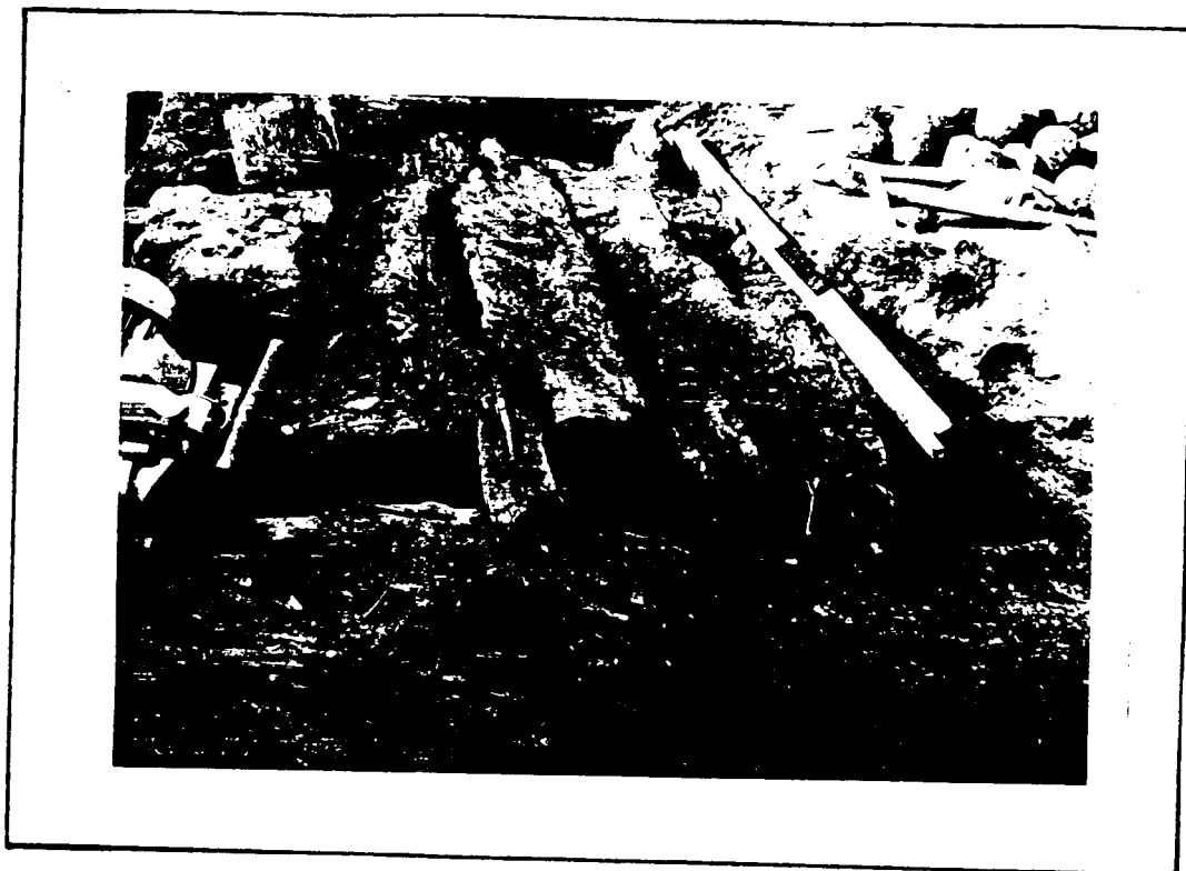
Figure 14g. Limber strake abutting keelson.
