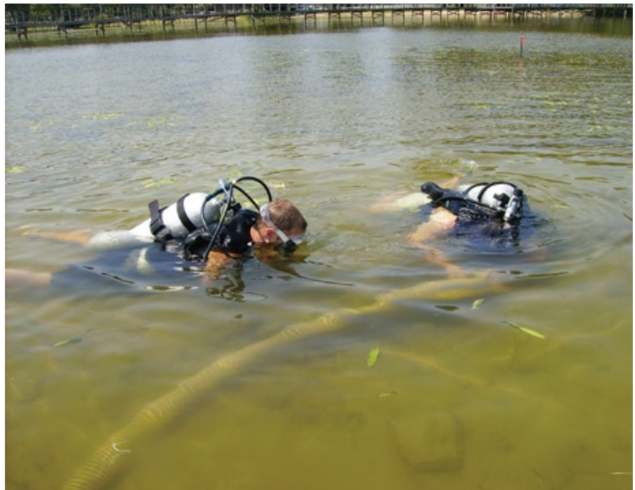
Dredging at boathouse site.
