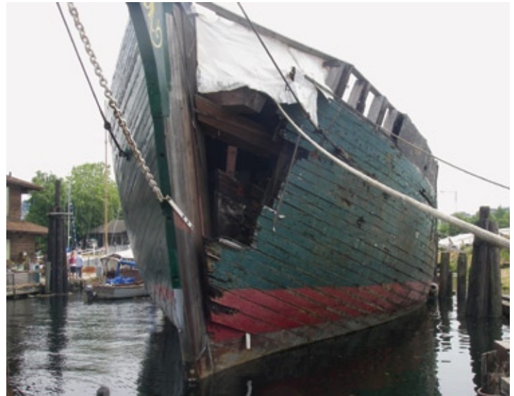
FIGURE 1: General view of Wawona ’s bow, showing gaping hole.
