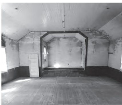
Reaves Chapel's interior, post demolition
