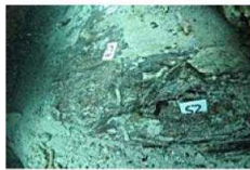
26-IMG_196-Scarf joint w planks numt
