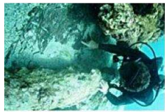
20-IMG_190-Overview scarf joint N of
