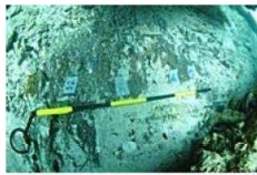
21-IMG_191-Scarf joint area N of C7 (w
