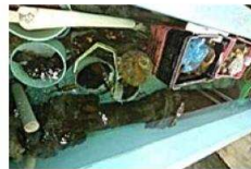
IMG_102-Conservation Tank Out
