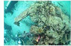
G_039-C pile C8 protruding +1
