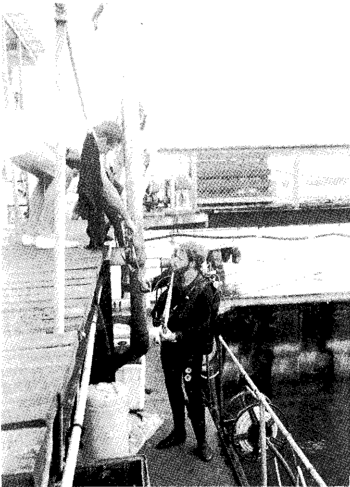
Working platform at the cofferdam
